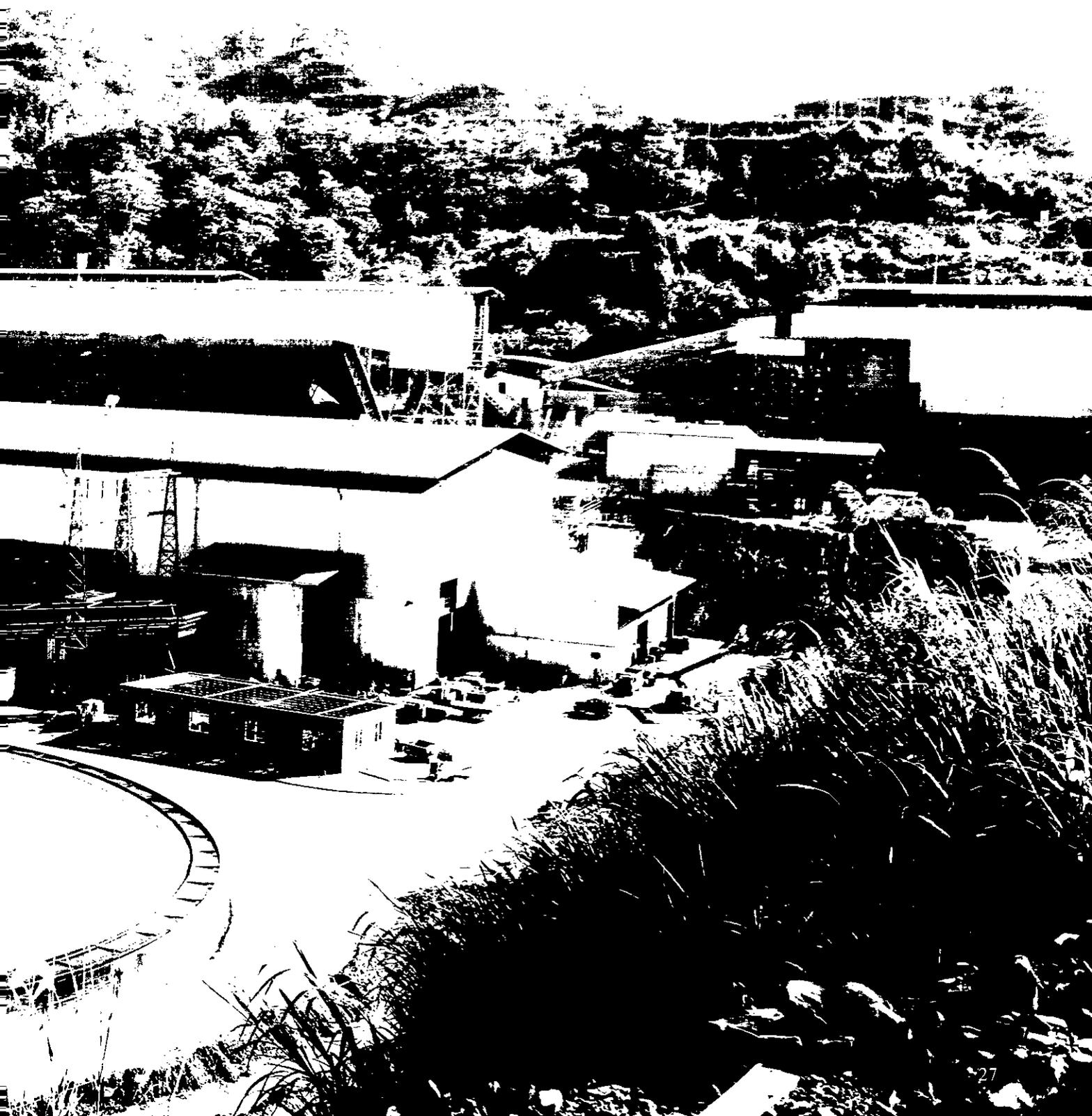
At the port site the slurry is filtered and dried to reduce the moisture content and the final concentrate product is stored ready for loading and shipment.
